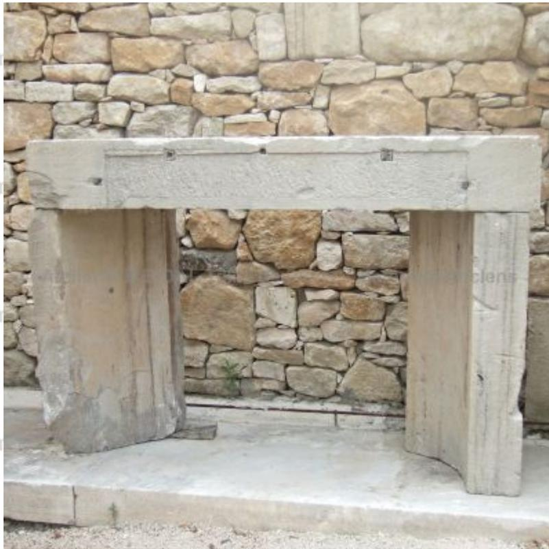
This antique limestone open-hearth cooking fireplace features a monolithic fireback and two molded jambs. Dating from the 19th century, this fireplace in stone also has 2 cast-iron stew holes, designed to be filled with embers for cooking.
